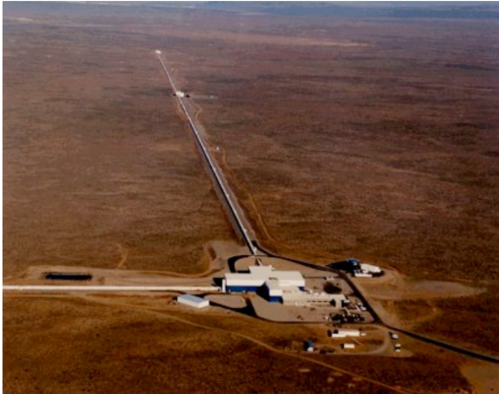
The LIGO facility in Hanford, Washington, showing one 2.5 mile arm, with the other arm going out of the picture to the left.
